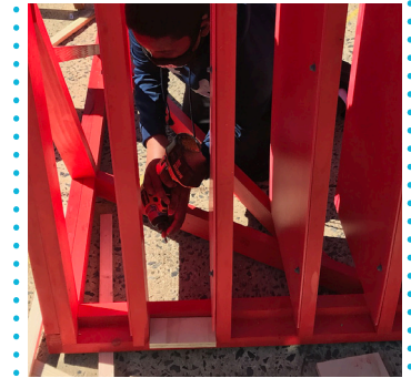
Attach with 2 ½" screws. Use 4 ½" blocks and work your way out to ends.
