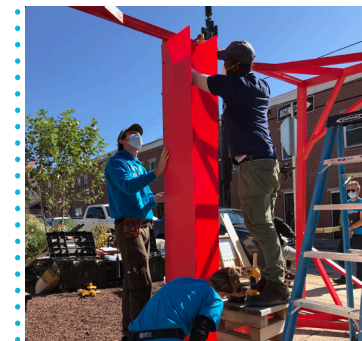
Begin installing shades from middle of structure. Screw from bottom.
