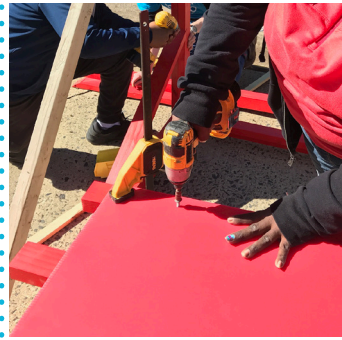
Assemble shades with coroplast sheets and 90° pressure treated rails.
