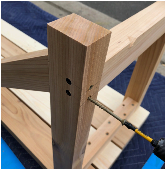
Attach with 3" screws.
