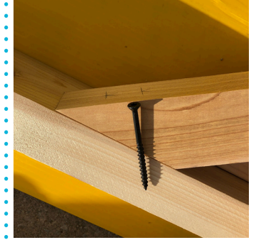
Hold a screw at the joint to determine what length to use to secure diagonal pieces.
