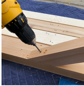
Attach 50° cut to seat slab. Double check that the seat and leg assembly are square.
