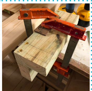
Using 2 1/2" screws, combine two 9 1/2" blocks together in an "L" shape. Remember to pre-drill.
