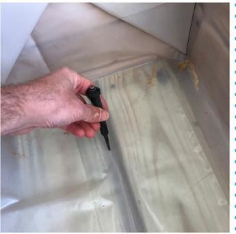
Pierce drainage holes into plastic along bottom between decking. About 6-8 holes throughout.
