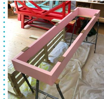
Assemble pine/ fir or cedar boards into two rings. Align and square all edges.
