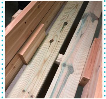
Lay the decking inside the ring, 1 ¼" from the edges. Attach with 1 ⅝" screws, 2 per plank, at each brace.
