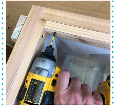
Attach ledger strips with 1 ⅝" screws. Remember to pre-drill.
