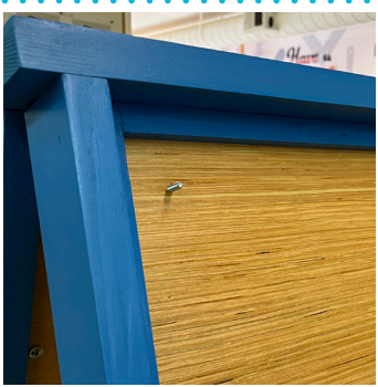
Thread the screw with the nut through the back of the plywood.
