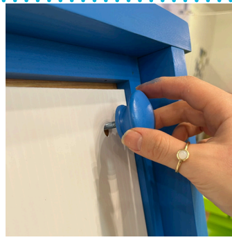
Place the coroplast signs in, and screw cabinet knobs in place.
