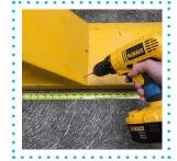
Have friend hold base in place, pre-drill and toenail 4 screws into each side of the seatboard
